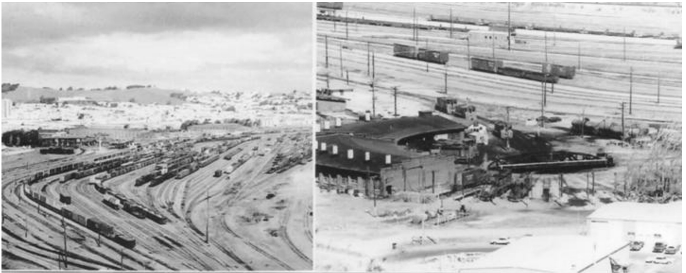
(LEFT) Looking northward at Bayshore Yard in 1962 we see many of the yard tracks with cars ready for movement. The tracks to the left were for departing trains; the tracks angling off to the right are arrival tracks. At left center is the roundhouse, sand tower, and shop buildings. (RIGHT) Looking down from San Bruno Mountain we see the 18 stall roundhouse and turntable. This was the second turntable installed here.
