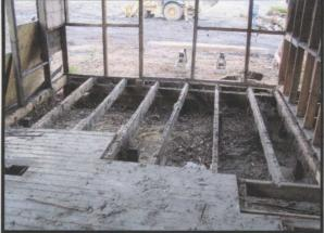
This view shows how easily we were able to remove the flooring. All the boards were held in place with square nails and some were nearly 14 feet in length. We removed all nails from all the wood before sorting and stacking.
