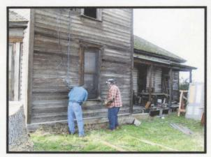
Bruce McGarvery (left) and John Powell (right) are removing the frame around one of the front windows. A few moments later they will begin removing the exterior wall siding that we will later use in restoring the old Woodville depot.
