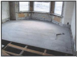
Jerry Hellinga is taking a short break after removing many of the long tongue and groove flooring. The floor joists underneath are full dimension lumber and in excellent shape. We removed all of these and, as you can see behind Jerry, quite a bit of the wall boards.
