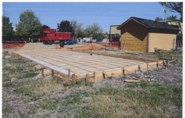
Jerry Hellinga and Ken Hill cut and laid the rebar late last month and now the foundation for the new library-archives building is ready for the pouring of concrete. It is hoped that the building would be finished before the summer season is over. — Tony Johnson photo
