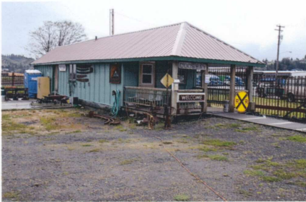
The headquarters for the Oregon Coast Chapter is this former storage shed, that was rebuilt to resemble a train depot. Located between the harbor and downtown Coos Bay, it is easy to find for first time visitors. — Tony Johnson photo
