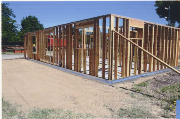
(RIGHT) From the other side of the building you can see the inner office walls. Notice the new metal flashing is in place and the trenched area around the foundation is now packed with decomposed granite. — Tony Johnson photo
