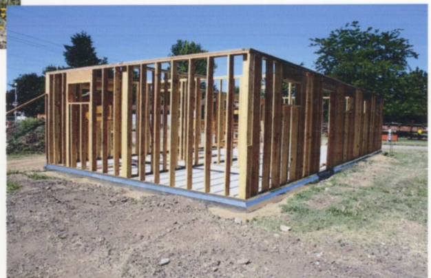
(RIGHT) From the other side of the building you can see the inner office walls. Notice the new metal flashing is in place and the trenched area around the foundation is now packed with decomposed granite. — Tony Johnson photo
