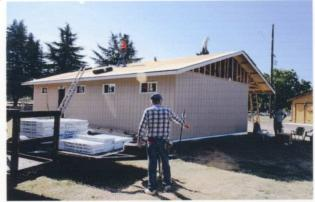
(LEFT) The roofing paper is nailed down on the south side; now it's time for the north. Chrisanne Murry is walking towards a roll of paper as Steve Bruff gets ready to load the chapter forklift with the bundles of shingles. Within an hour of this photo the temperature climbed to over 90 degrees... and it wasn't 11:00am yet! — Tony Johnson photo
