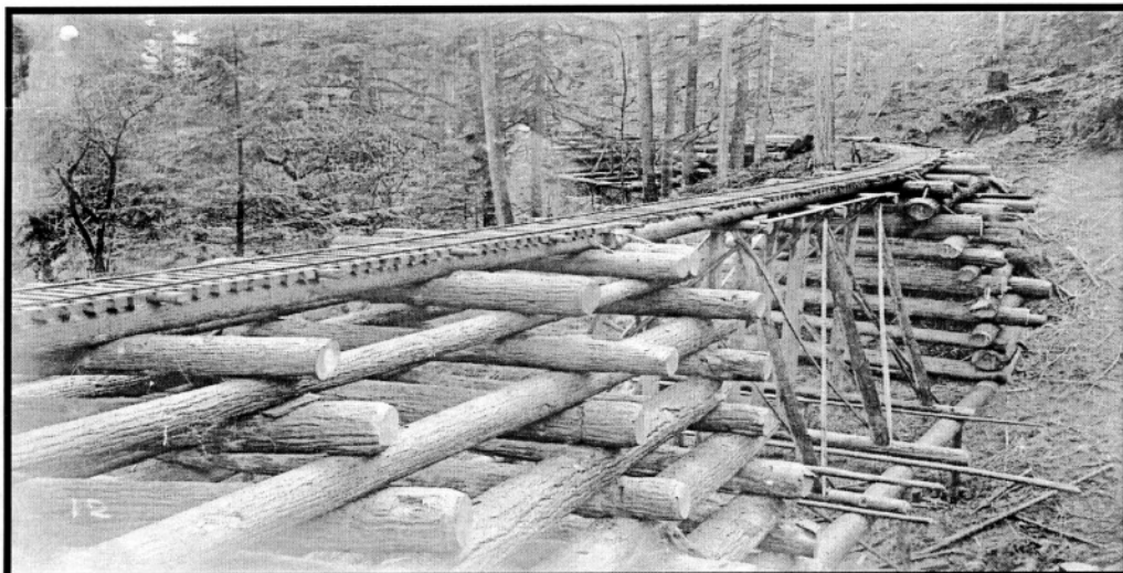
Combination of intermittent cribs and conventional trestle in this section
