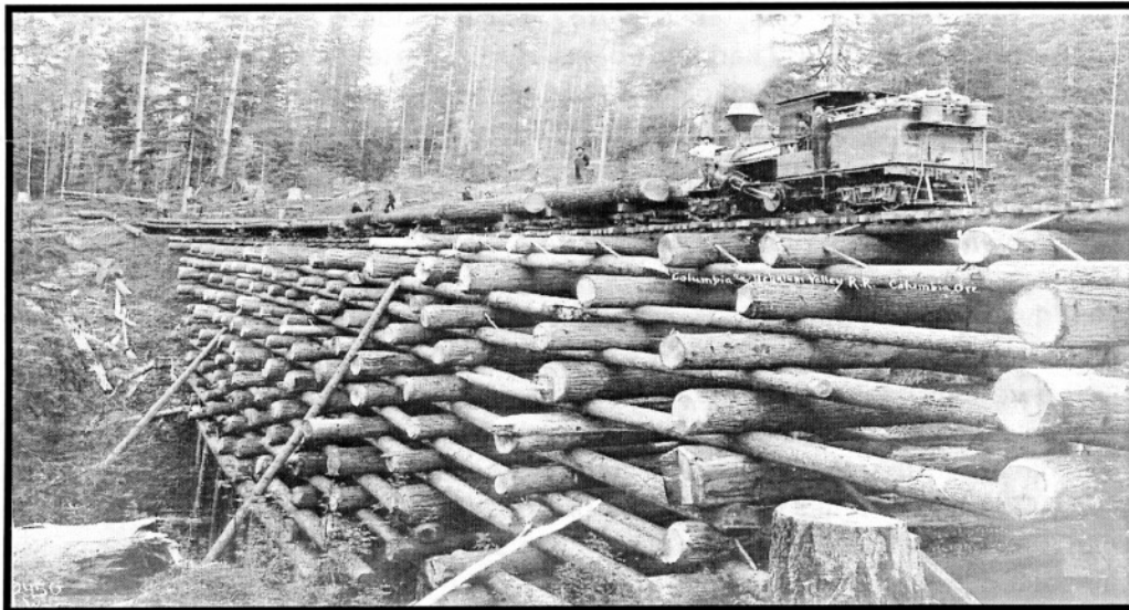
Combination of intermittent cribs and conventional trestle in this section
