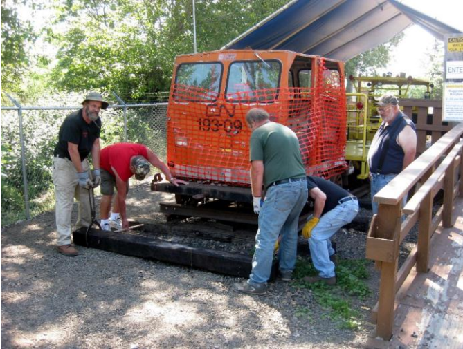
First New tie being laid by the crew. Rick Aubin Photo
