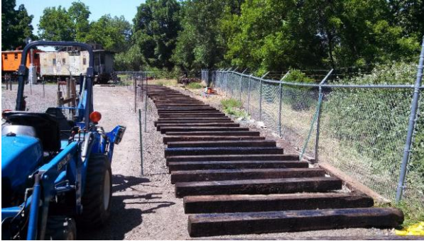
The newly laid ties. Rick Aubin photo
