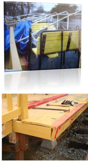
The call went out for ditch diggers to begin excavation for a concrete base on both sides of the platform. These would house the support posts for the new roof. Actually, modern equipment (blue color) was hauled to the work site and would facilitate the preparatory work. Only a few (human) ditch diggers volunteered. In the meantime, new 2x6 decking planks replaced the buckling platform. A coat of SP company paint added to the fresh look of the station.
