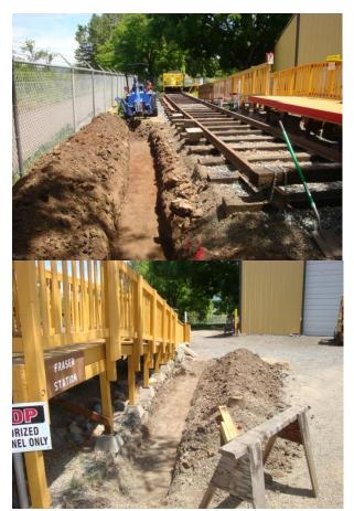
In preparation for the concrete footing, the ditch digger gets a lot of the credit. The forms were made via the group method with plenty of sweat equity all around.
