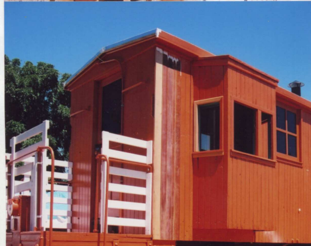
[LEFT] Steve wasn't happy with a few of the end boards so he worked on them as well. After these photos were taken, Steve applied the Elastomeric caulking in between the seams on every board on the flanger. This should prevent any moisture from penetrating behind the paint. He'll then give the entire flanger another primer coat and several finish coats of orange.
