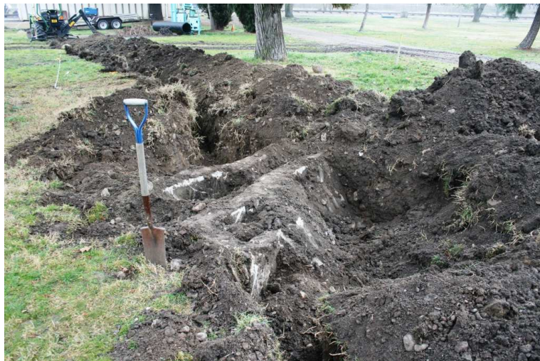
(RIGHT) While we may have had our problems finding buried concrete while digging our trenches; the Live Steamers had a tough go of it, too. It may be difficult to see in this photo, but next to the shovel is a three ring wall of concrete, reinforced with rebar. After jack-hammering the first portion to trench level, Jerry found stenciled markings showing 30 inches, meaning there was more than 30 inches more of concrete underneath.
